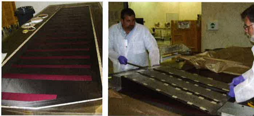
Figure 5. Left – Film adhesive (FM@209-1K) strips for I-beam flanges; Right – Locating aluminum filler blocks with back-to-back C-channels to make I-beams.
